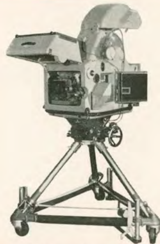
Studio type Technirama camera showing new blimp with the various doors open giving access to the camera for lens change, re-loading, etc.
